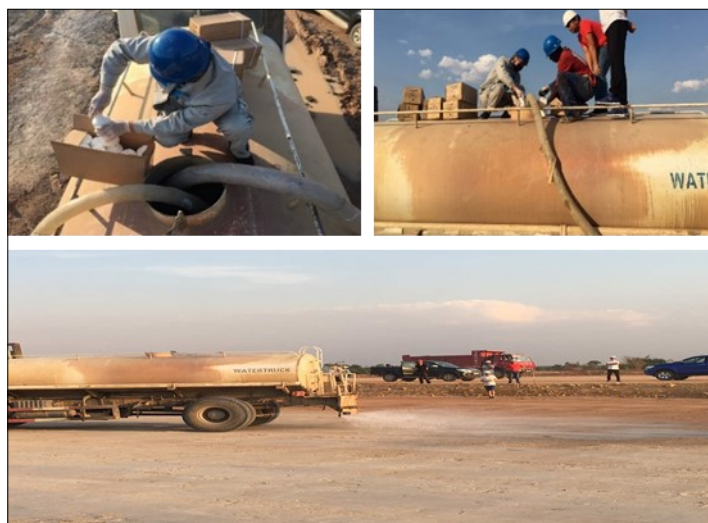
Fig. 8. The mixing of chemicals and spraying with a tanker at site
