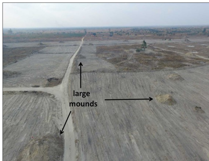
Fig 3. Aerial view assessment of mounds spreading over the construction site
